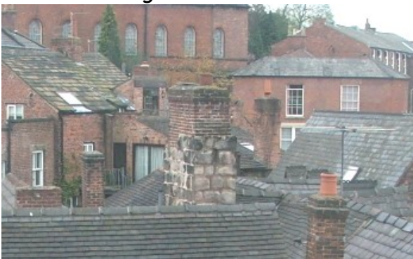
Medieval Chimney Stack
